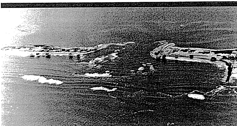
Figure 21. The Westhampton barrier breached during the December 1992 northeast storm forming Little Pike's Inlet in Moriches Bay. (Photo: First Coastal Corp)
