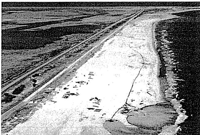
Figure 26. Inlet bypassing and beach nourishment project on Jones Beach Island. Sand dredged from Fire Island Inlet (in the background) is piped to the site and deposited on the shoreline to build a beach to protect the Ocean Parkway. (Photo: American Dredging Company)
